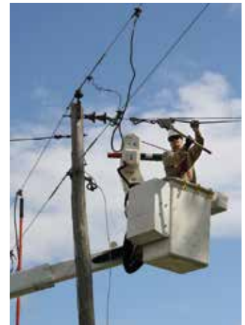
After a storm, ACEC line crews identify which damaged lines to work on first based on which lines will restore power to the greatest number of members.
