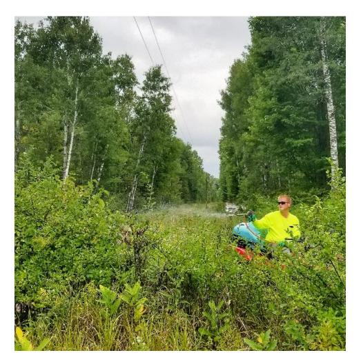
Our line clearing contractor will carefully and accurately apply herbicides to those areas in the overhead power line right-of-way where trees and underbrush are beginning to reappear.
